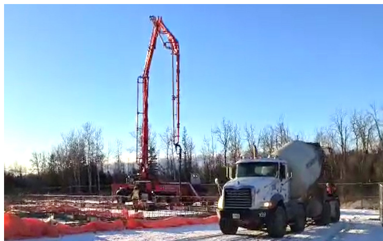
December 2024, the first truck with concrete arrives!
